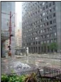
Glass from broken office windows, downtown Houston
