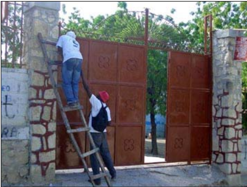
The completed front gate
