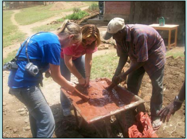
Kayo and Aurora helping mix the red concrete finish
