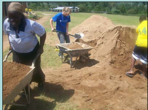
Moving the cement to the classroom
