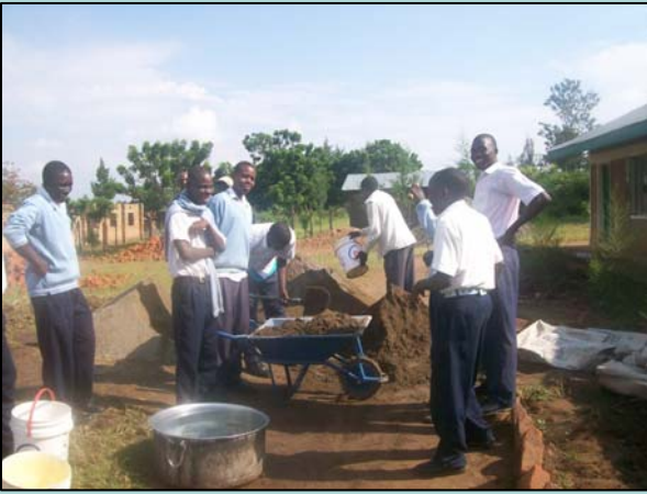
Mixing the cement
